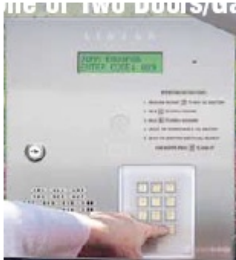
Figure 2. Picture of the telephone entry system.
